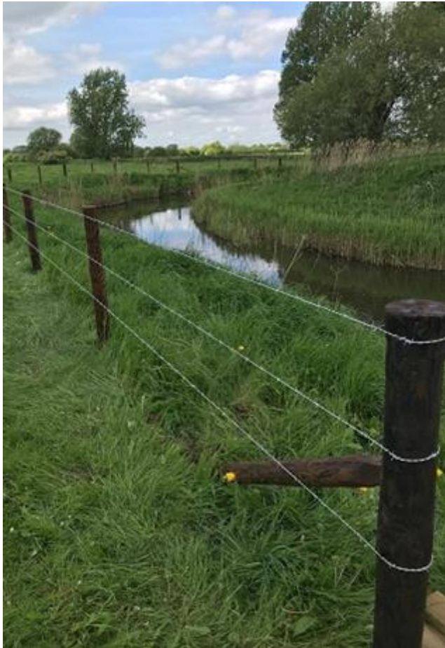
Figure 4 New fencing installed at Elton
