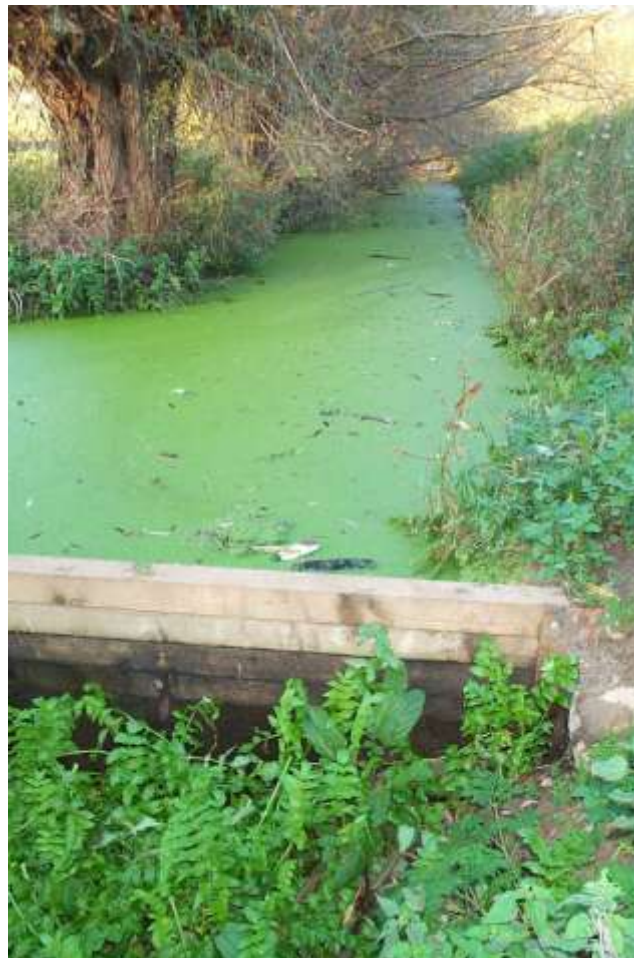
Photo 5 A seepage barrier
