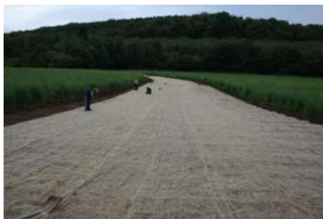
Photo 3 Grassed waterway under construction
