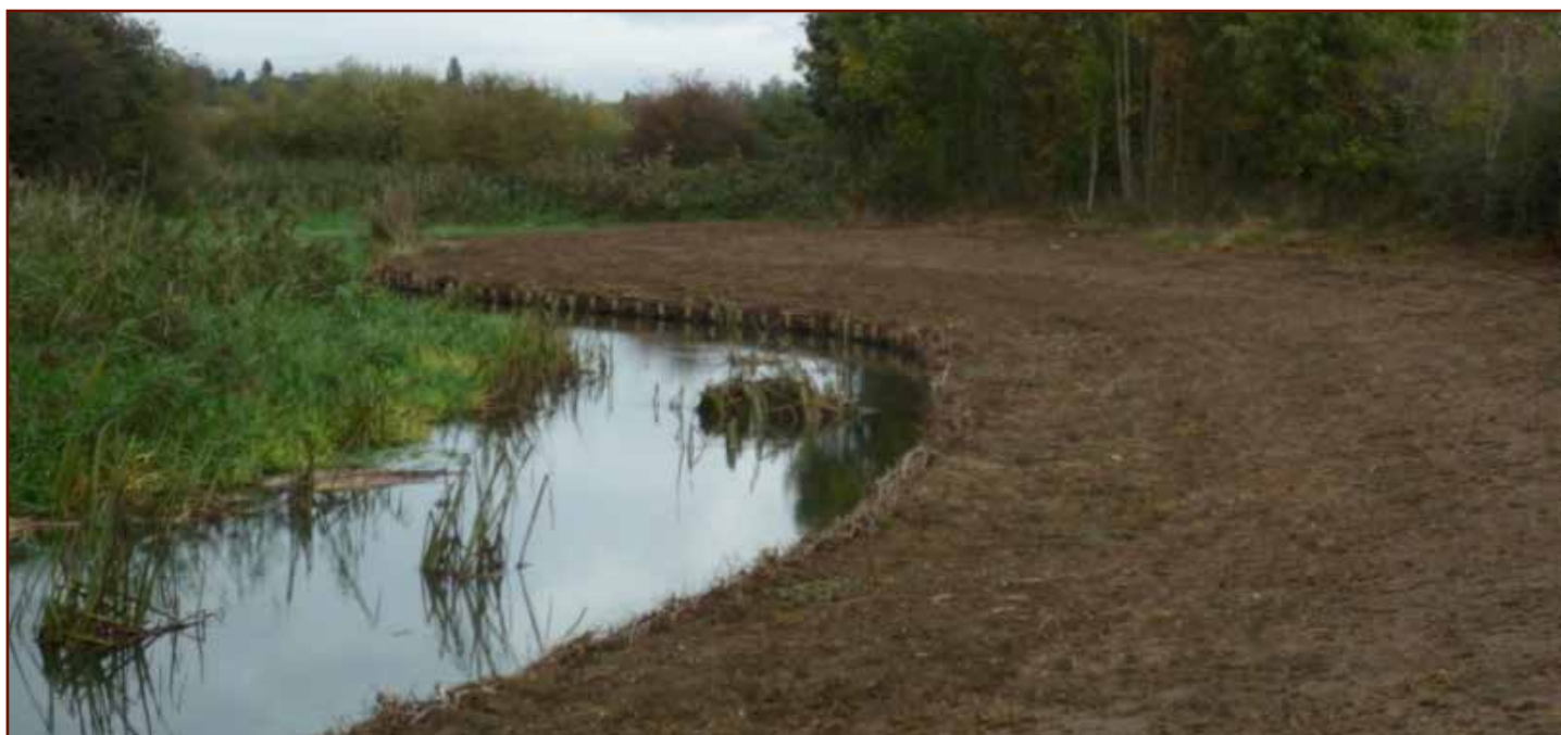
A section of the River Nene that has been re-landscaped and narrowed at Duston Mill. Vegetation will soon appear on the bare bank.
