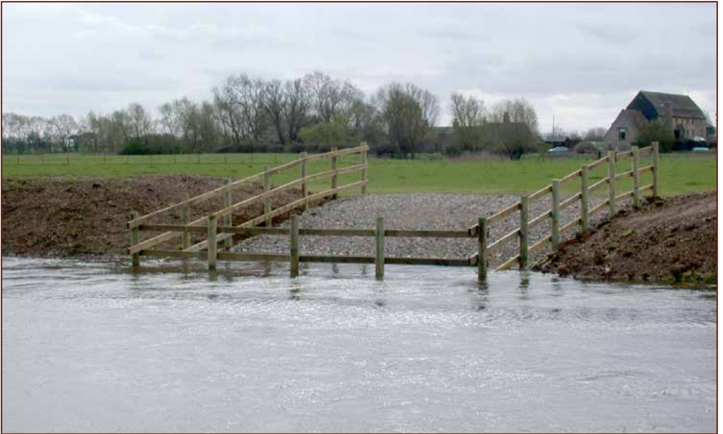
A cattle-drinker on the Castor Back Channel of the River Nene, to the west of Peterborough. Note the stone lining on the ground. (Photo: © R. S. Brayshaw Ecological Consultancy)
